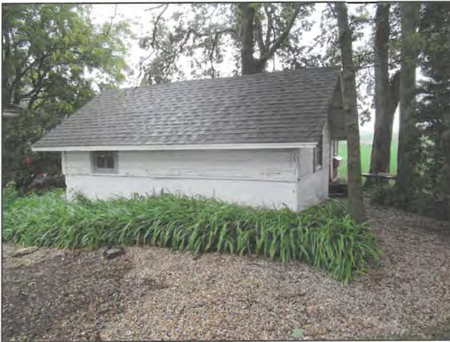
Photograph 20: View of Resource 09d, camera facing east.
