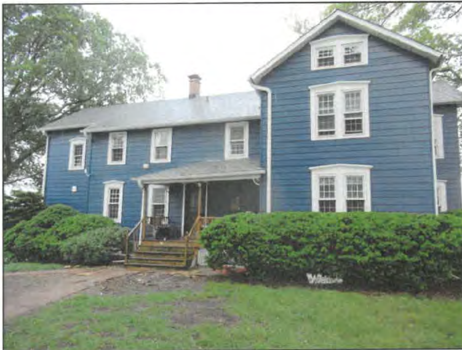
Photograph 6: View of Resource 09a, camera facing south.
