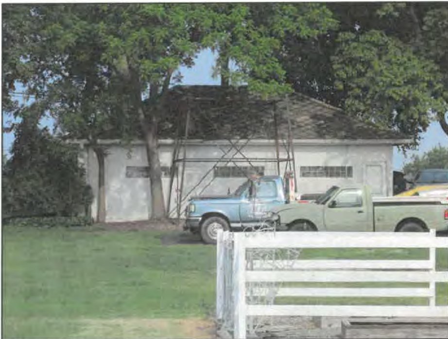
Photograph 16: View of Resource 09c, camera facing west.
