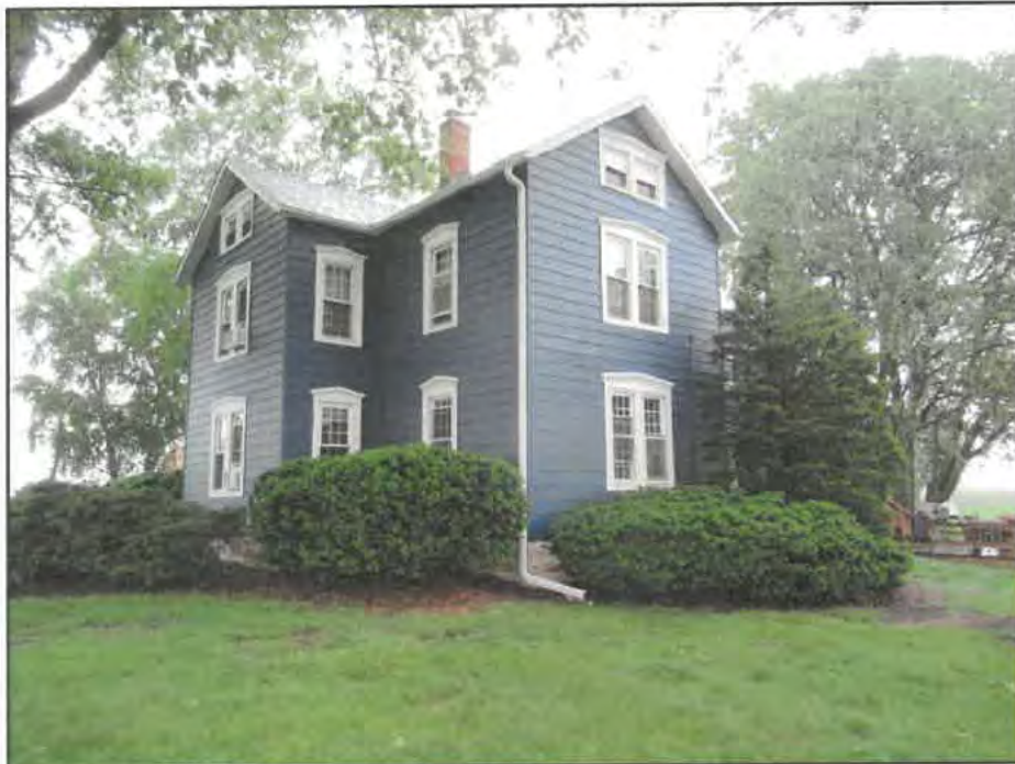
Photograph 4: View of Resource 09a, camera facing northeast.
